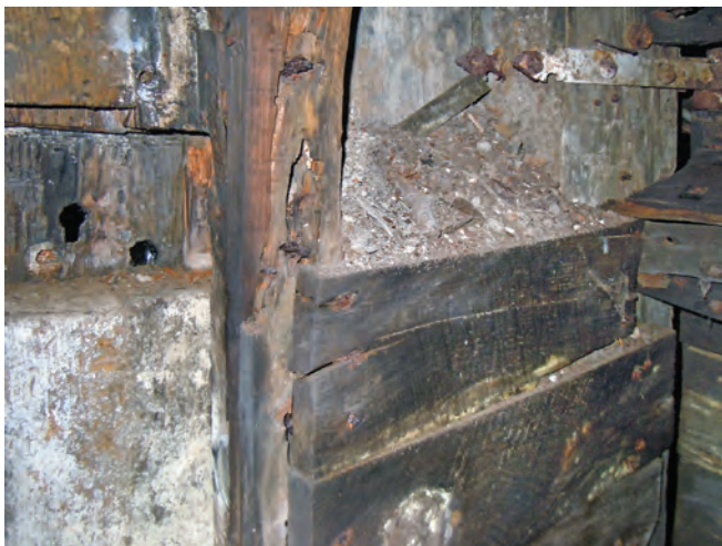
Inside view of the blast door
